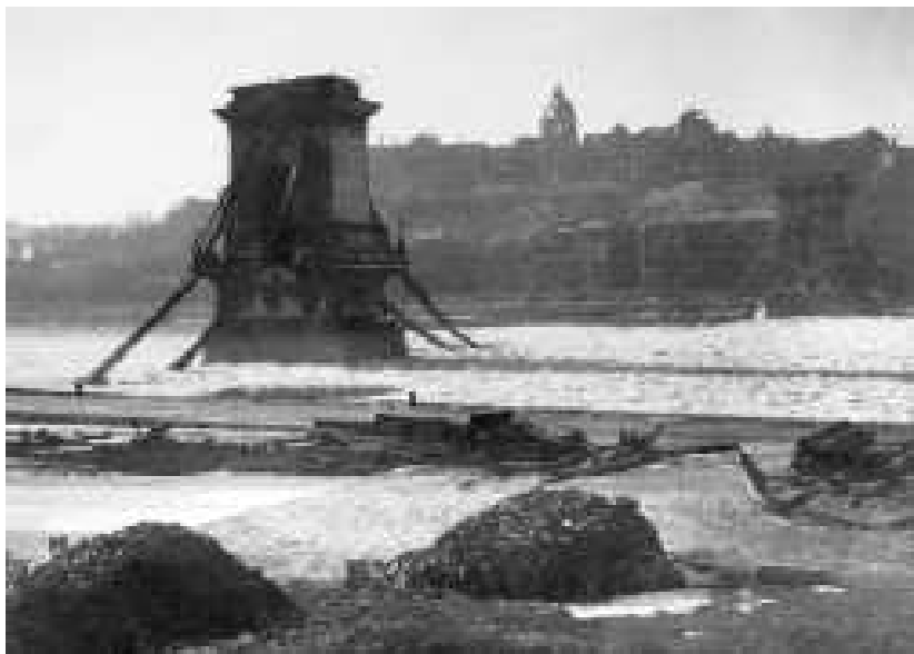
Lánchíd (Chain Bridge) blown up at end of WWII, photo by id. Takács István
