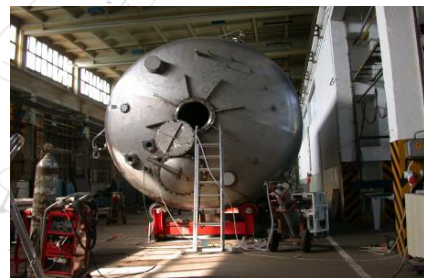
On-site special leak testing
